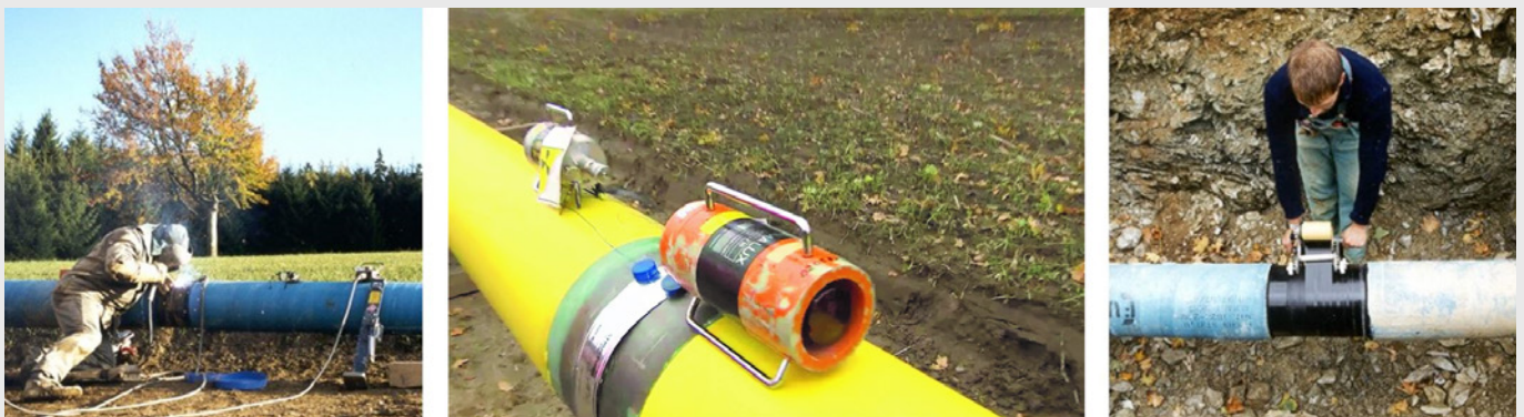
Figure 1: Welding, testing and field coating
